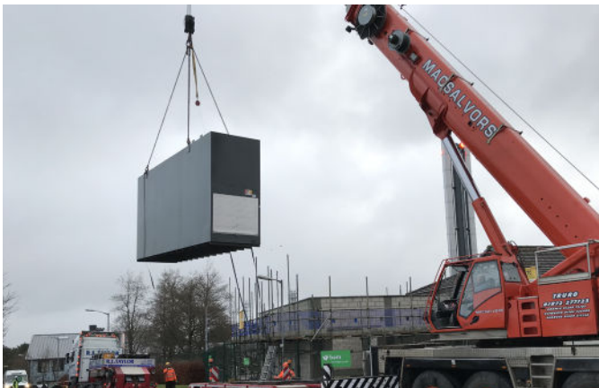
The 56,000 storage tanks arrive on-site and are lifted into position
