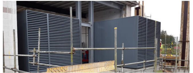
The outlet attenuators are moved into positioned into the plant room
