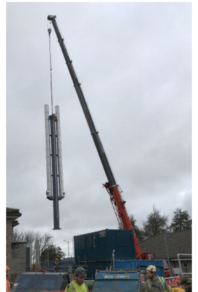
The exhaust flues are craned into position and installed on-site at the hospital
