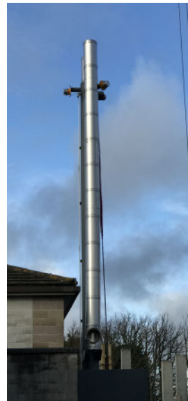
The exhaust flues are craned into position and installed on-site at the hospital
