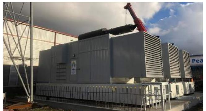
The installed generating sets positioned on top of the three 45,000 banded belly day tanks
