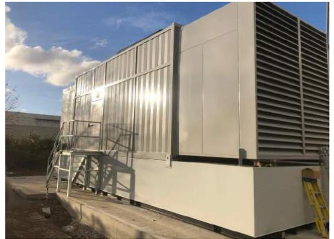
The generators in position on-site, within acoustic containers, built with additional access steps due to the containers being sat on the belly tanks
