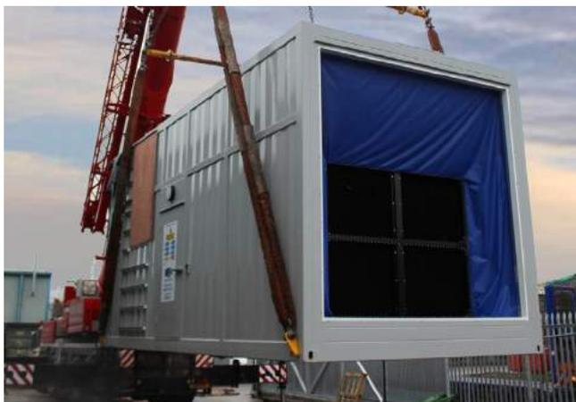
One of the T1900 Generators being lifted onto a Hiab after FAT testing at WB Power's Derbyshire facility
